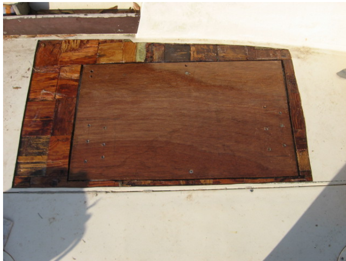
Figure 6 New core plate in position with countersunk screws and epoxy.
