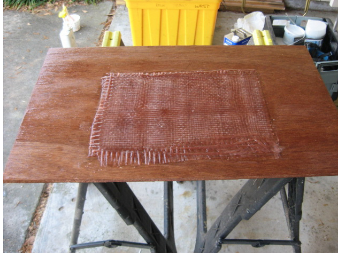
Figure 3 Roving was used to make a backing plate
