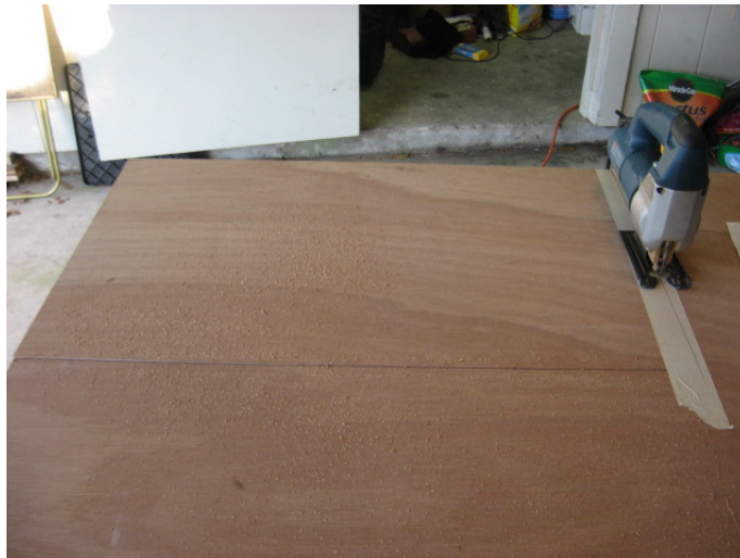
Figure 2 Use masking tape on crosscuts to minimize splintering
